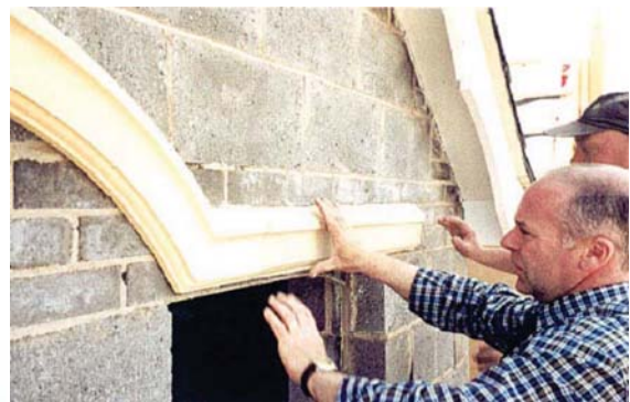
PHOTO 2 - FINAL UNIT IN PLACE
