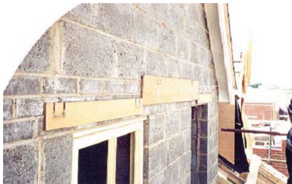
PHOTO 1 - TIMBER TEMPLATES IN PLACE
