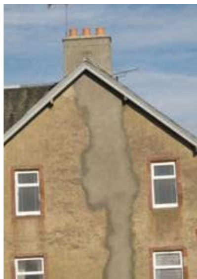
A flue relined from the outside.
